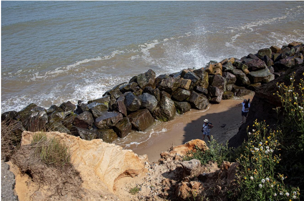
Image 24 Rock Armour clearly dissipating wave strength at Happisburgh Alan D Horn Aug 2020
